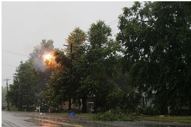
Tree limbs create a short circuit during a storm, typically resulting in a power outage
